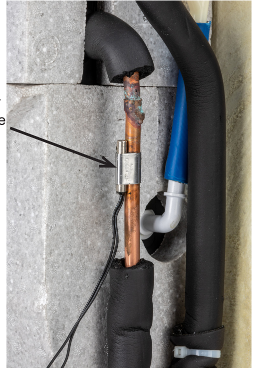
Water Temperature Thermistor Location
